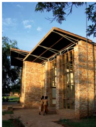
Figure 3: Ndere Centre, Kampala
