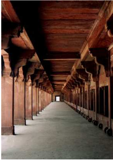
Figure 9. Stable showing Traditional Indian Trabeated System.
